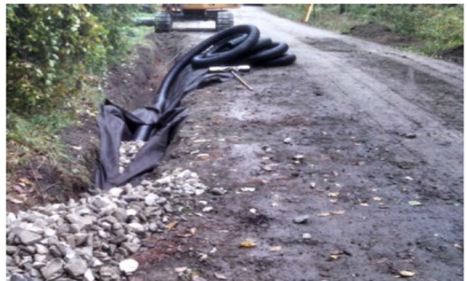
The ditch above was always wet from roadside springs. This underdrain will collect spring flow to keep the roadbed and ditch dry.
